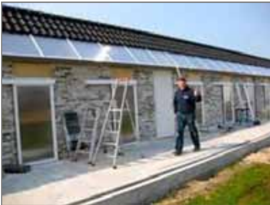
New lofts under construction
